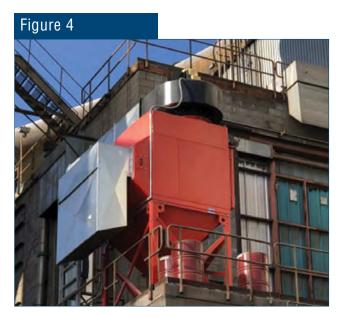
Self-maintaining air cleaner installed on exterior of steel mill.
